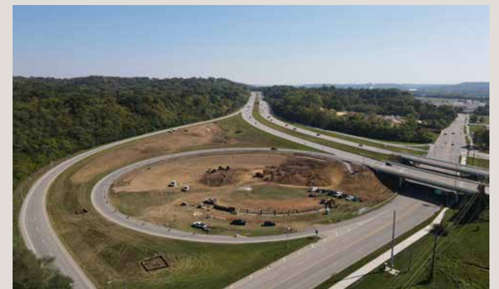
Gateway improvements to the Interstate 275 interchange started this fall.
